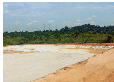
Ground improvement site (Gelang Patah, 2017)
